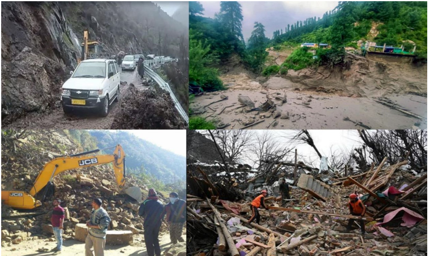
Fig. 8 Field photos from the Kulgam and Anantnag Districts survey showing rock formations and landslides caused by poor rock mass conditions
