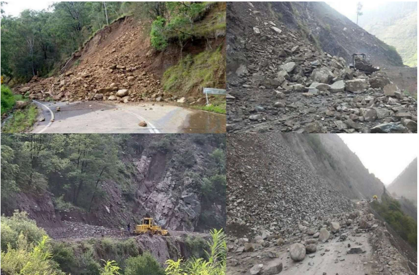
Fig. 5 Field photos from the Ganderbal Sonmarg Road survey showing rock formations and landslides caused by poor rock mass conditions
