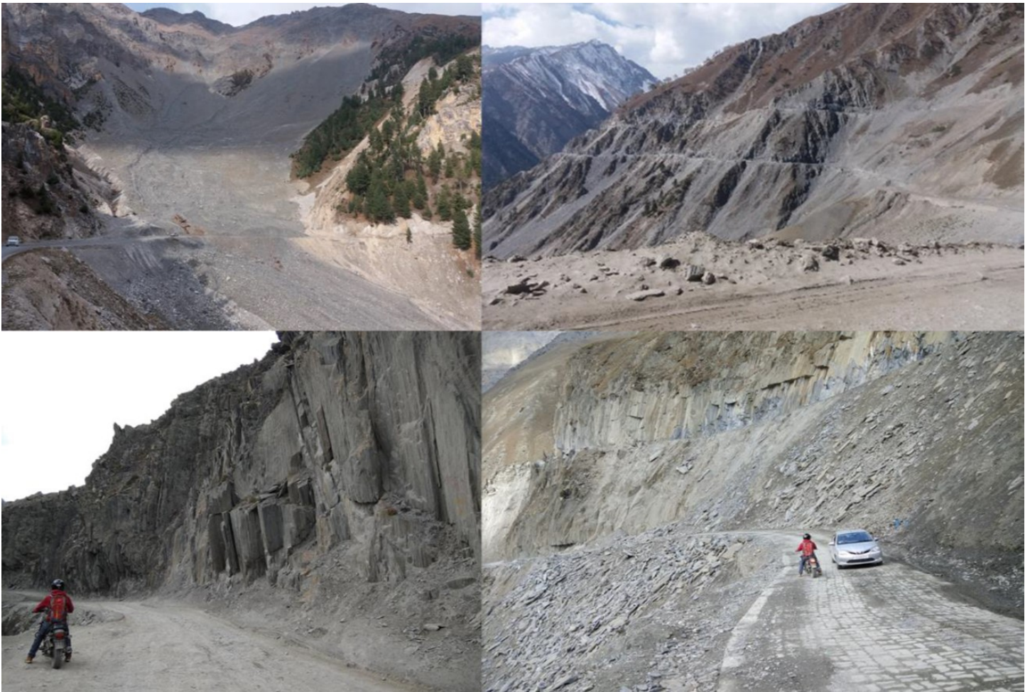
Fig. 6 Field photos captured during geological survey along the Zojila Pass road, showcasing the diverse rock formations
