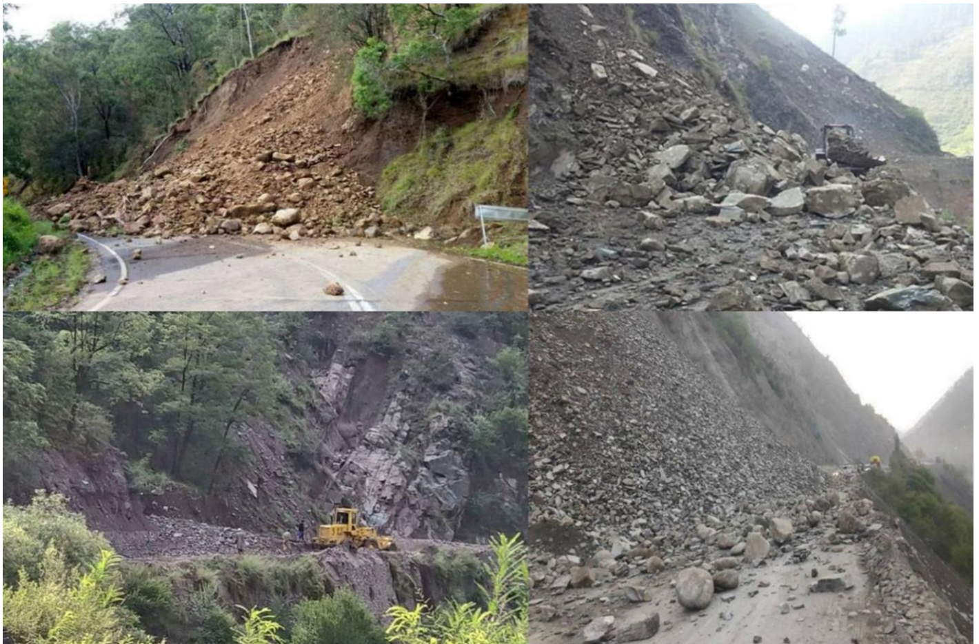
Fig. 3 Field photos from the Baramulla-Uri Road survey showing rock formations and landslides caused by poor rock mass conditions
